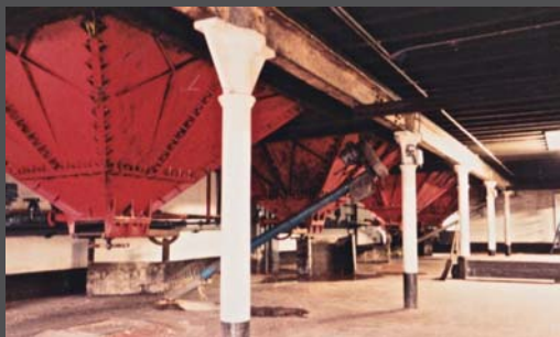
Steeps (tanks) for soaking the barley
